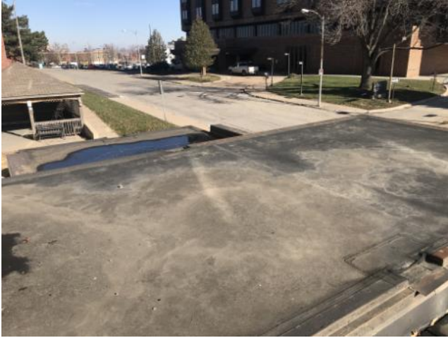
Roof Overview Section 5
