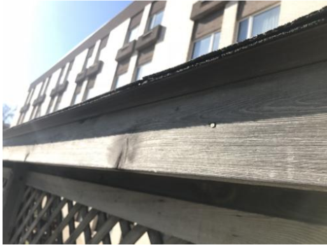
Wood Fascia In Good Condition
