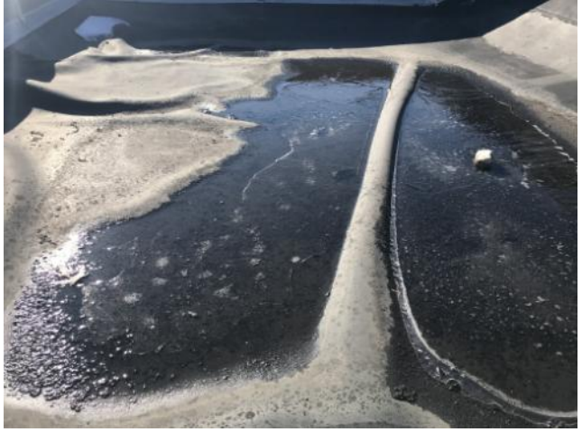
Scupper Flashings Starting To Fail
