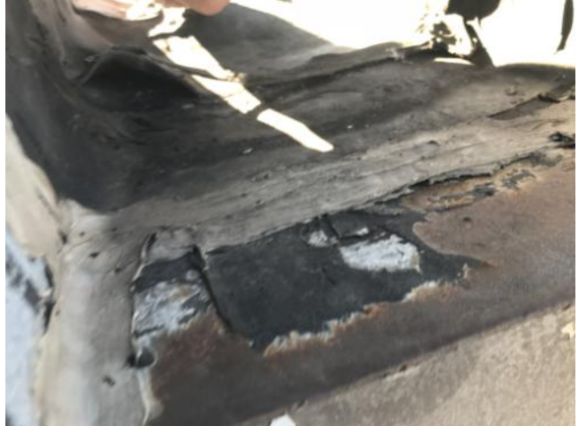
Scupper Flashings Starting To Fail
