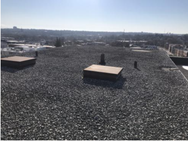
Roof Overview Section 2
