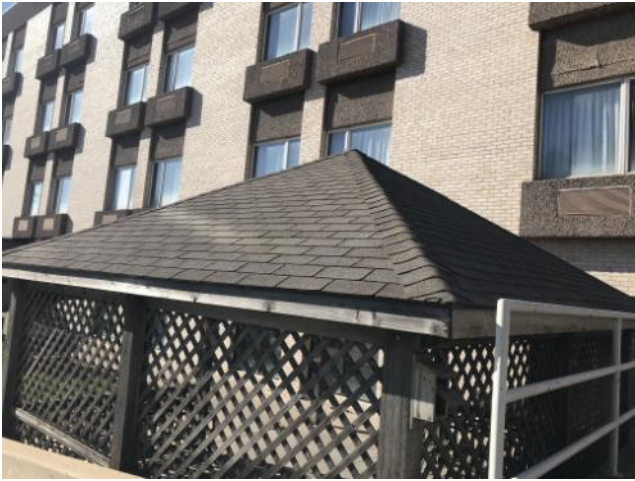
Roof Overview Section 6
