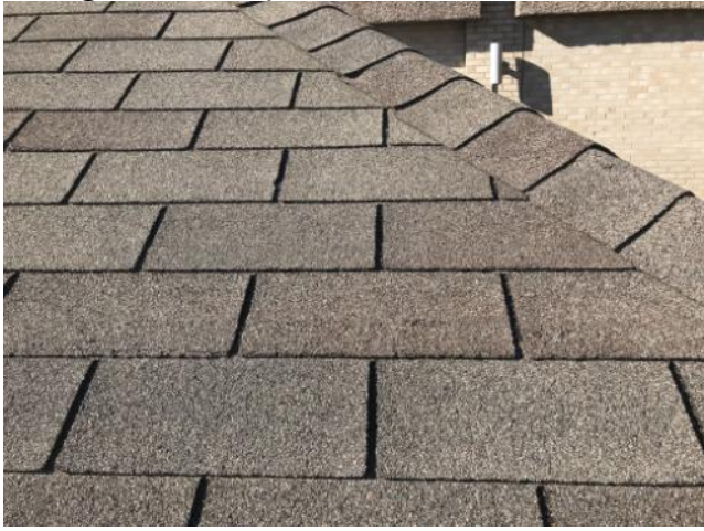
Shingles In Acceptable Condition
