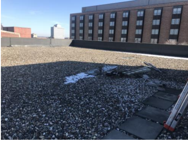
Roof Overview Section 1
