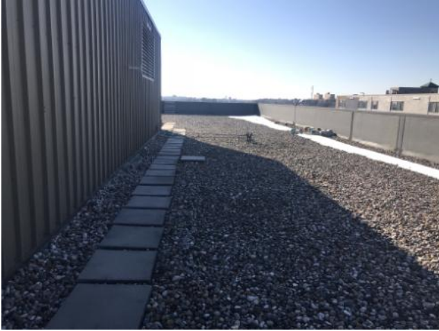
Roof Overview Section 1
