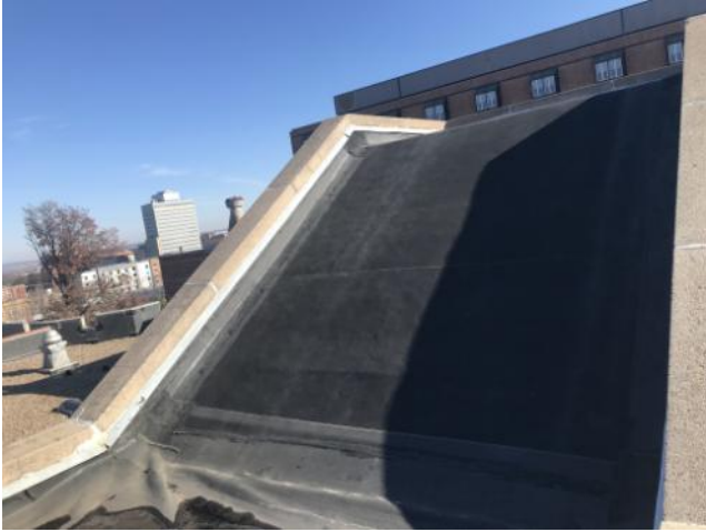
Roof Overview Section 3
