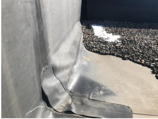
One Run Of Heavy Pulling (15')
