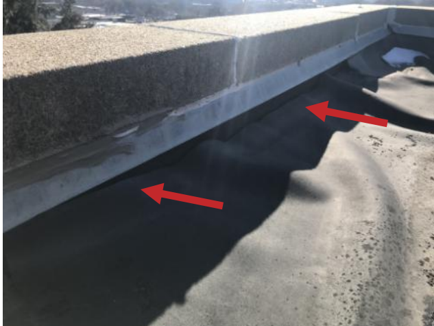
Wide Open Run Of Flashing (6')
